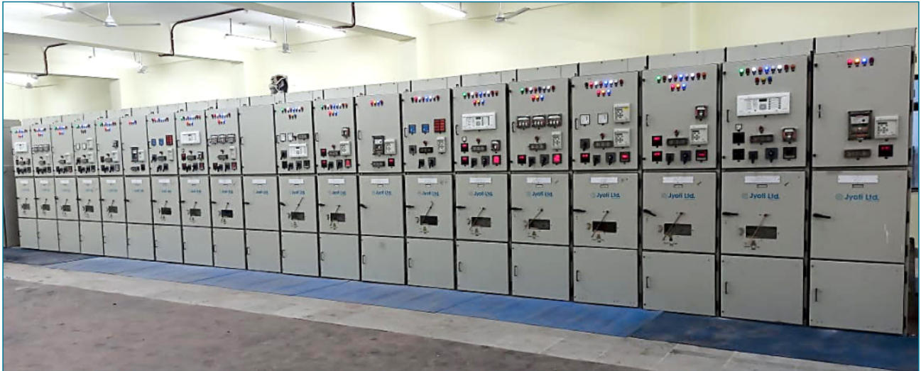
HT VCB Panels for IOCL Pipeline Division at Jamnagar Gujarat.
